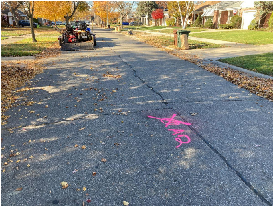
Photograph No. 2: Low to moderate severity transverse and longitudinal cracking with crack sealing near boring A-2. View to the west.
