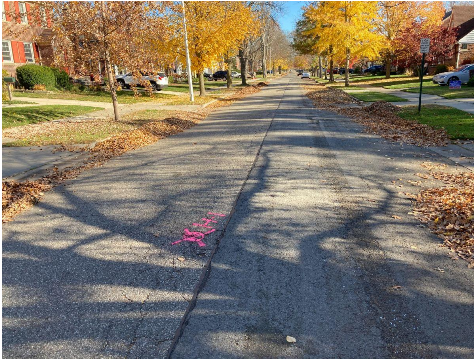
Photograph No. 7: Moderate severity transverse, fatigue and longitudinal cracking with crack sealing and full depth replacement patching along Hampton Road near boring H-1. View to the east.
