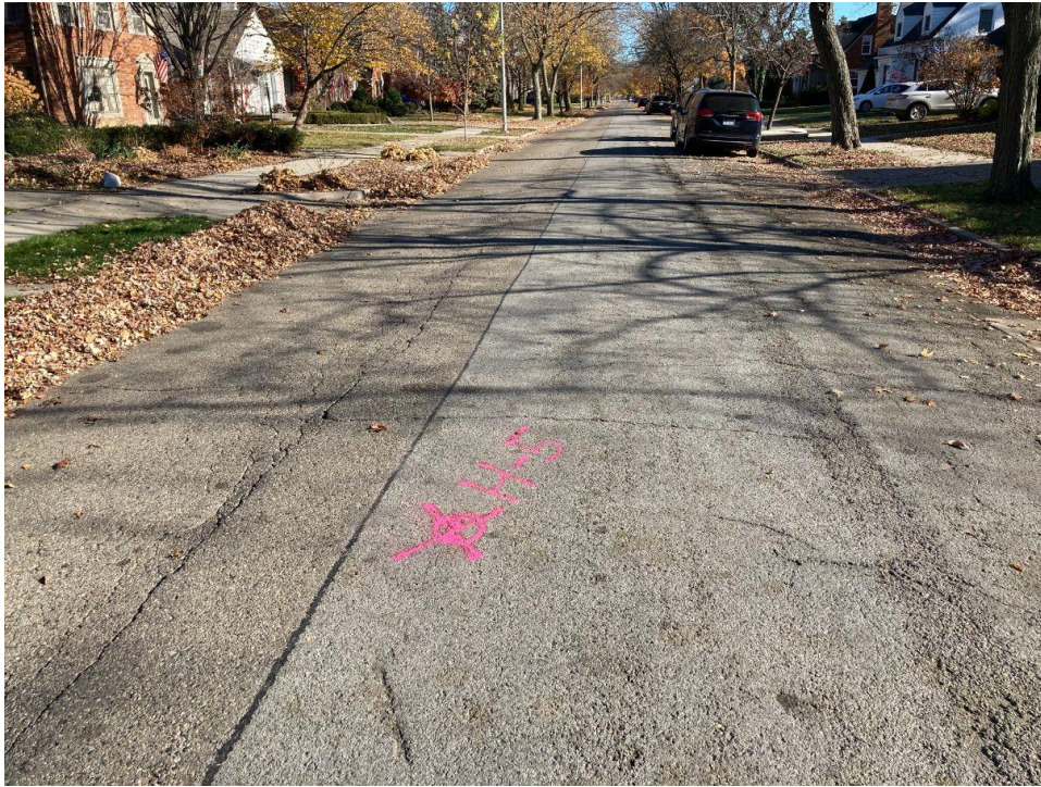
Photograph No. 11: Moderate severity transverse, fatigue and longitudinal cracking with full depth replacement patching and crack sealing along Hampton Road near boring H-5. View to the east.
