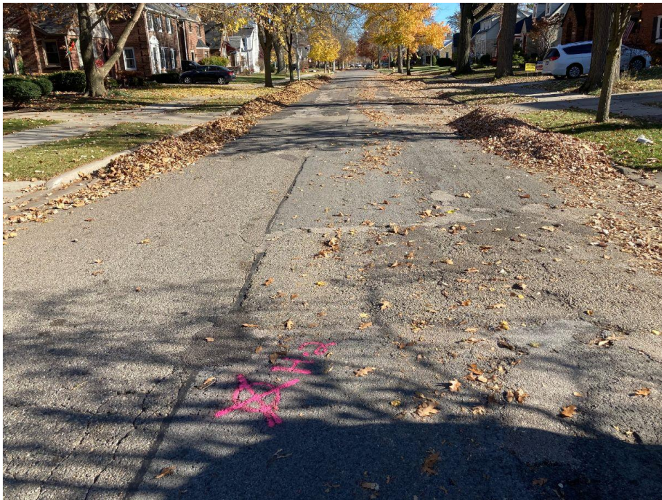
Photograph No. 8: Moderate severity transverse, fatigue and longitudinal cracking with cold patching, crack sealing, and full depth replacement patching along Hampton Road near boring H-2. View to the east.
