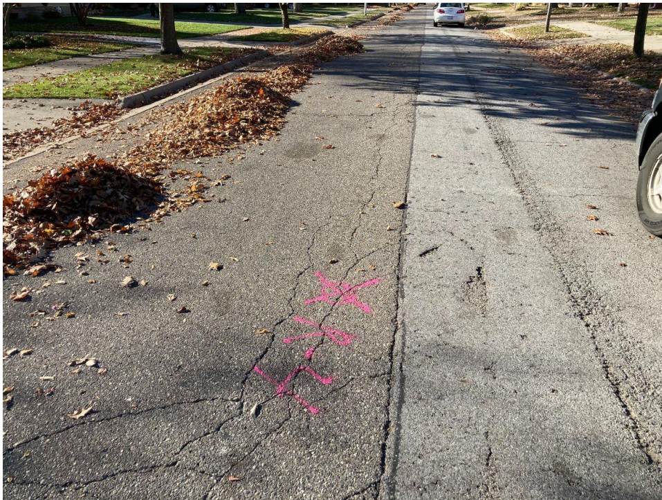
Photograph No. 16: Moderate severity transverse, fatigue and longitudinal cracking with crack sealing and full depth replacement patching along Roslyn Road near boring R-4. View to the west.
