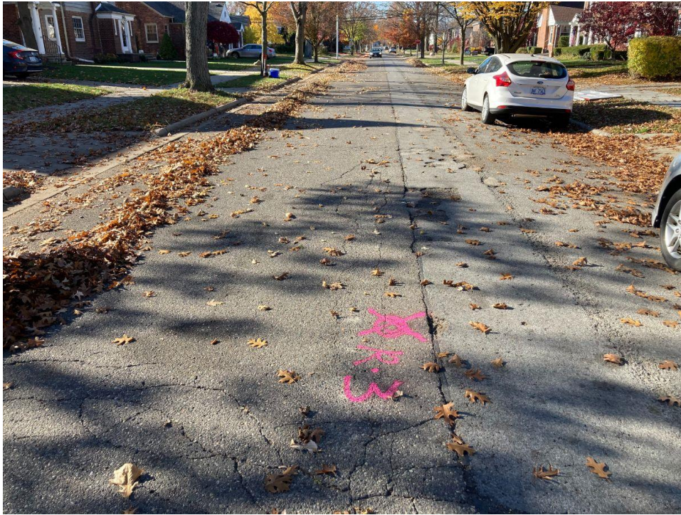
Photograph No. 15: Moderate severity transverse, fatigue and longitudinal cracking with crack sealing and full depth replacement patching along Roslyn Road near boring R-3. View to the west.
