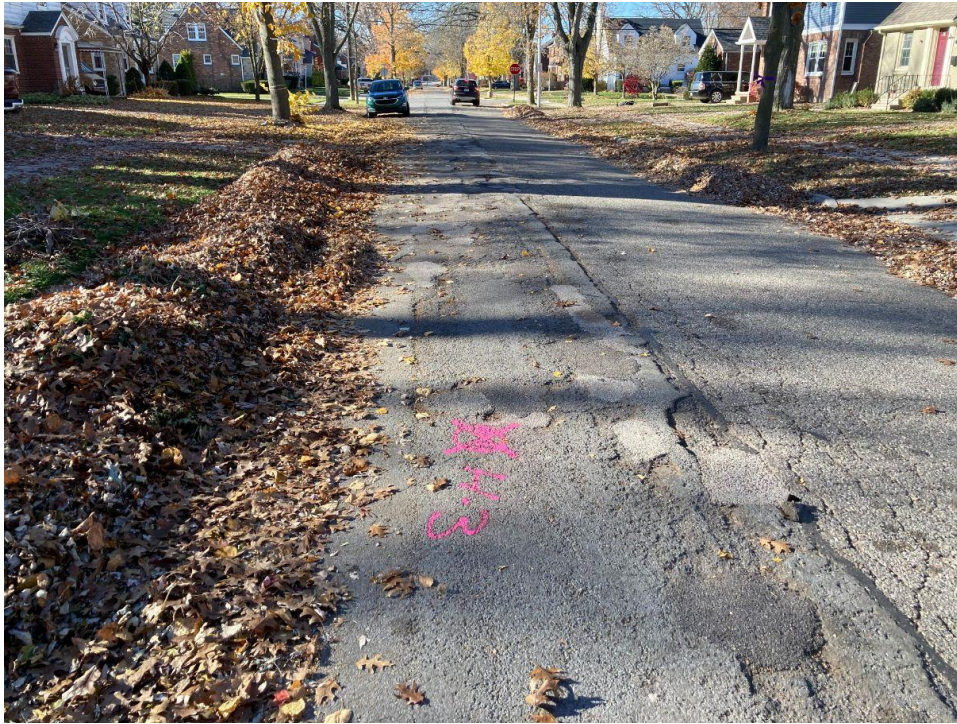
Photograph No. 9: Moderate to high severity transverse, fatigue and longitudinal cracking with cold patching, crack sealing, and full depth replacement patching along Hampton Road near boring H-3. View to the west.
