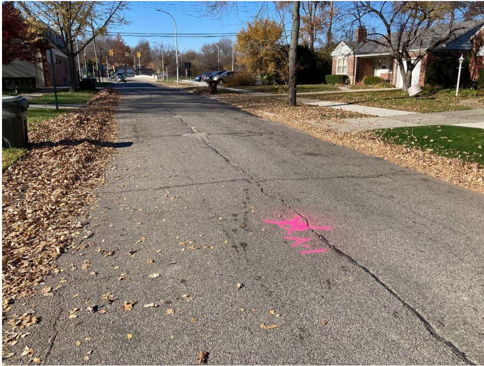
Photograph No. 1: Low to moderate severity transverse and longitudinal cracking with cold patching near boring A-1. View to the west.
