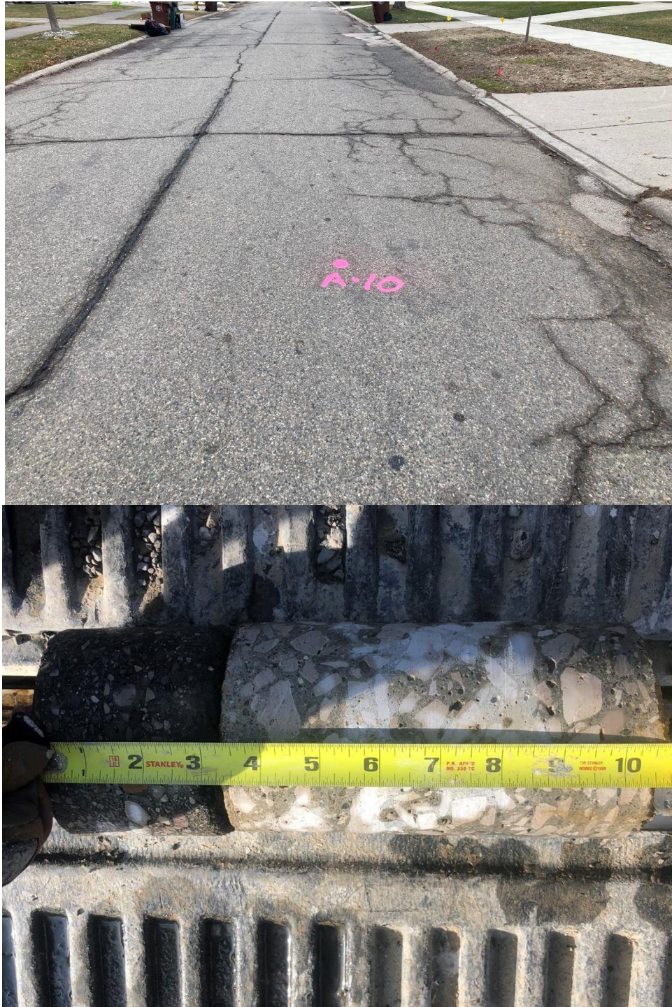
Photograph No. 10: Moderate severity transverse and longitudinal reflective cracking with cold patching near boring A-10. View to the west. Note the underlying Portland cement concrete contains limestone aggregate.
