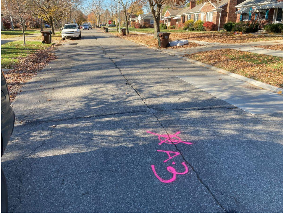
Photograph No. 3: Low to moderate severity transverse and longitudinal cracking with cold patching and full depth replacement patching near boring A-3. View to the west.
