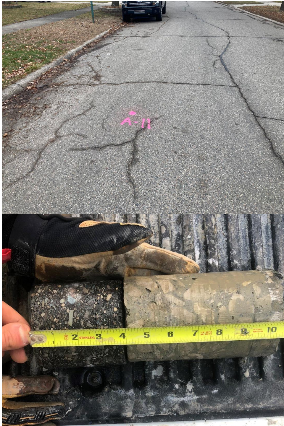
Photograph No. 11: Low to moderate severity transverse and longitudinal reflective cracking with cold patching near boring A-11. View to the west. Note the underlying Portland cement concrete contains limestone aggregate.
