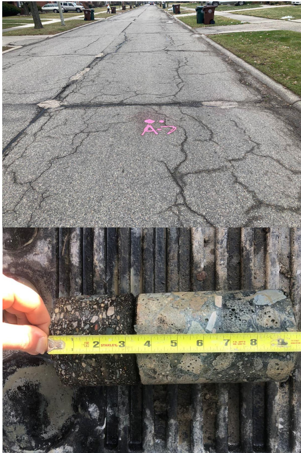
Photograph No. 7: Moderate to high severity transverse and longitudinal reflective cracking and edge cracking with cold patching near boring A-7. View to the east. Note the underlying Portland cement concrete contains slag aggregate.
