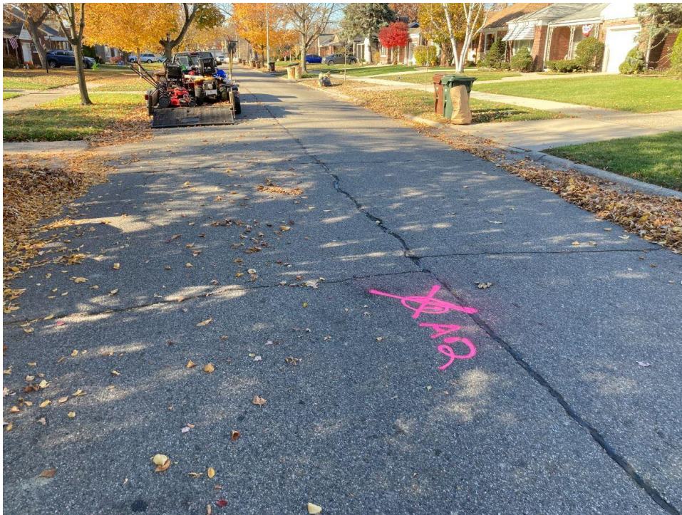
Photograph No. 2: Low to moderate severity transverse and longitudinal cracking with crack sealing along Allard Avenue near boring A-2. View to the west.
