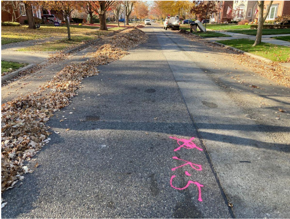
Photograph No. 17: Moderate severity transverse, fatigue and longitudinal cracking with crack sealing and full depth replacement patching along Roslyn Road near boring R-5. View to the west.
