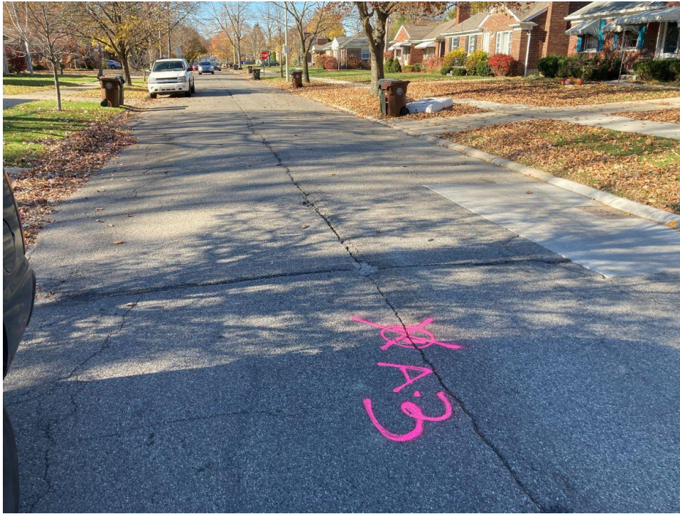
Photograph No. 3: Low to moderate severity transverse and longitudinal cracking with cold patching and full depth replacement patching along Allard Avenue near boring A-3. View to the west.
