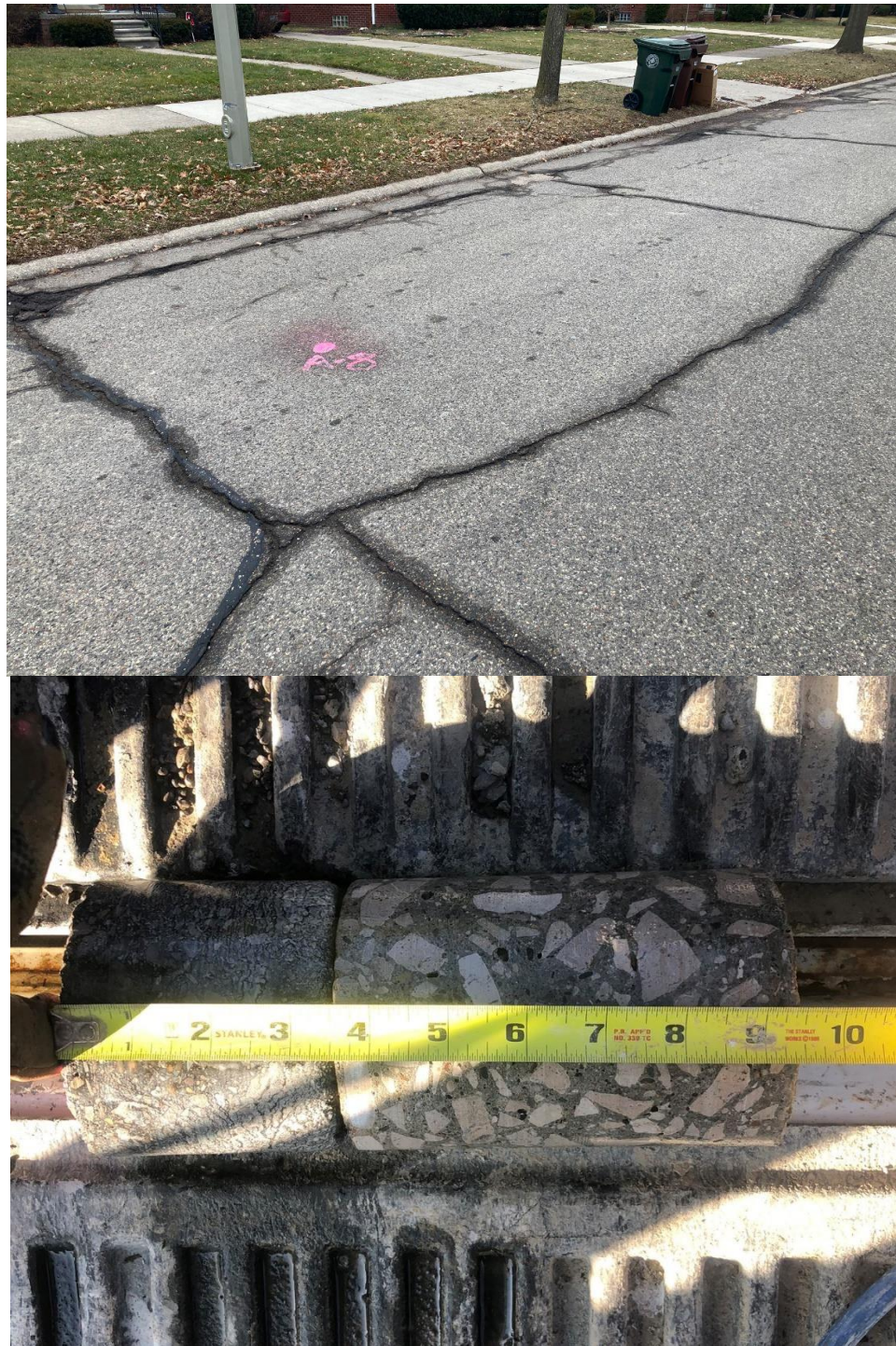
Photograph No. 8: Moderate severity transverse and longitudinal reflective cracking and edge cracking with crack sealing near boring A-8. View to the northeast. Note the underlying Portland cement concrete contains limestone aggregate.
