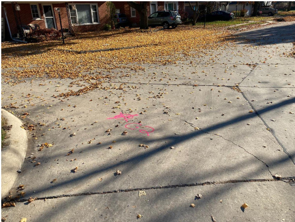
Photograph No. 6: Moderate severity transverse and joint cracking with crack sealing along Christine Court near boring C-2. View to the south.
