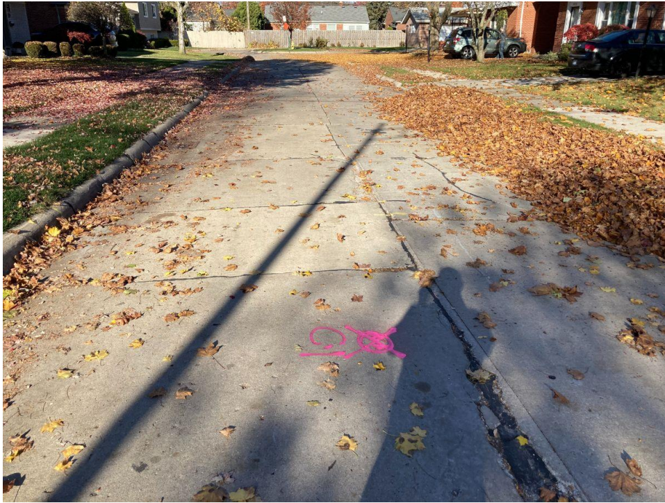
Photograph No. 5: Moderate severity transverse and joint cracking with crack sealing along Christine Court near boring C-1. View to the north.
