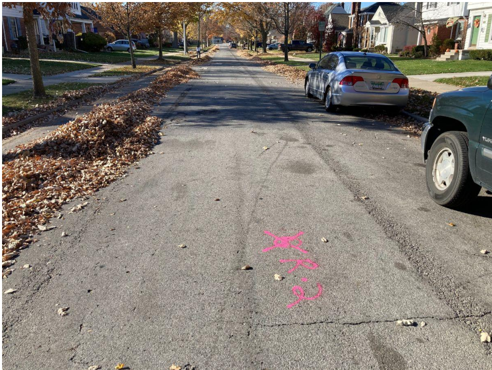
Photograph No. 14: Low to moderate severity transverse, fatigue and longitudinal cracking along Roslyn Road near boring R-2. View to the west.
