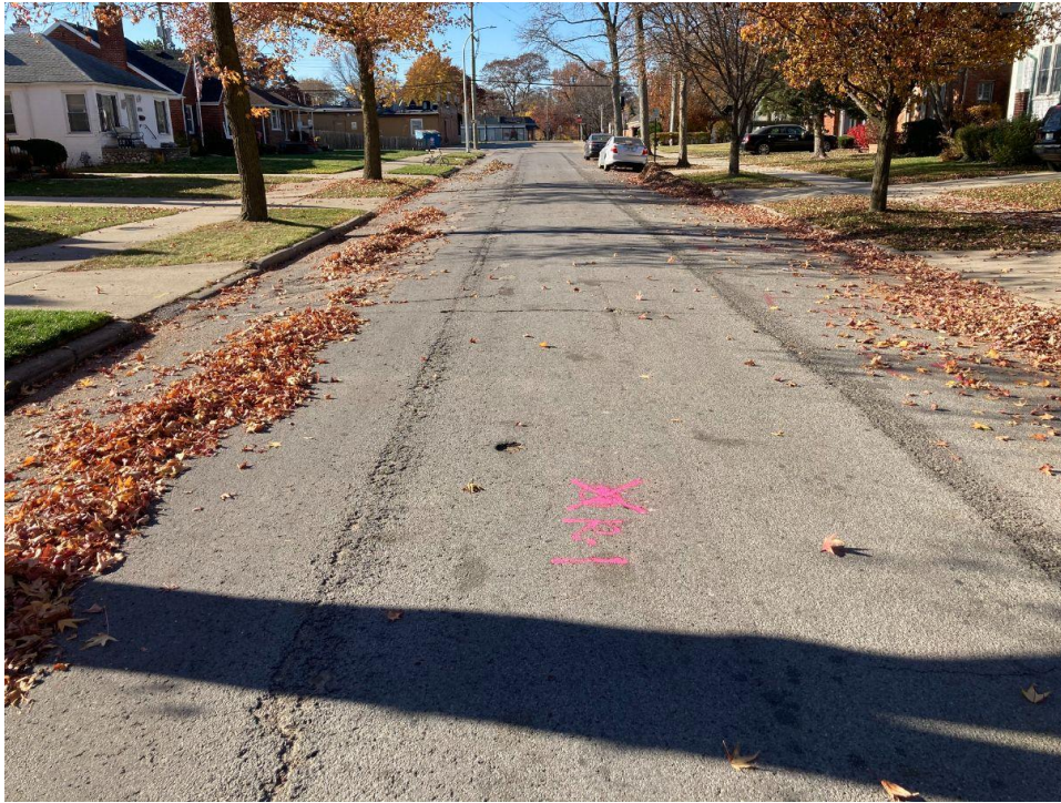
Photograph No. 13: Low to moderate severity transverse, fatigue and longitudinal cracking along Roslyn Road near boring R-1. View to the west.
