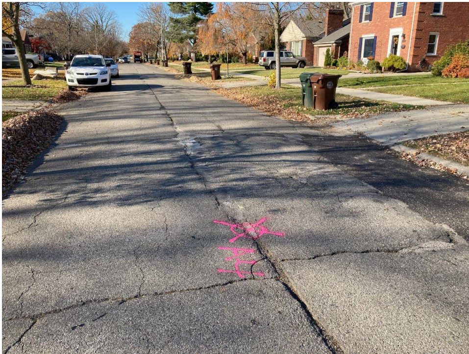
Photograph No. 4: Moderate severity transverse and longitudinal cracking with cold patching and full depth replacement patching near boring A-4. View to the west.
