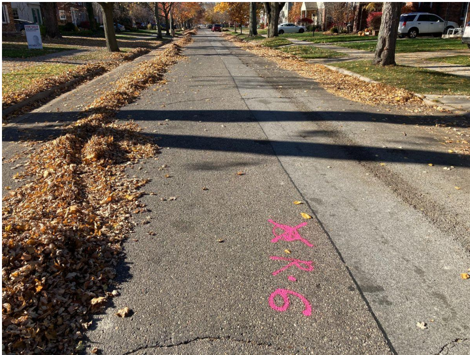
Photograph No. 18: Moderate severity transverse, fatigue and longitudinal cracking with crack sealing and full depth replacement patching along Roslyn Road near boring R-6. View to the west.
