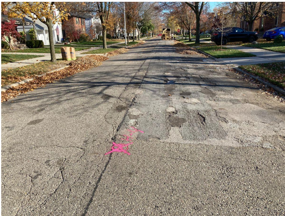
Photograph No. 10: Moderate to high severity transverse, fatigue and longitudinal cracking with cold patching and crack sealing along Hampton Road near boring H-4. View to the east.
