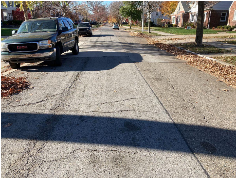
Photograph No. 12: Moderate severity transverse, fatigue and longitudinal cracking with full depth replacement patching and crack sealing along Hampton Road near boring H-6. View to the west.
