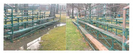
The bleachers on all the fields have become broken down. Caution tape was placed where boards were broken, damaged or completely removed. We would also be interested in upgrading the base of the bleachers to eliminate the flooding and unsafe conditions around the area when it rains.
