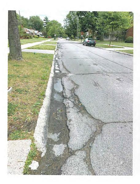
Nearly every curb is damaged, making it difficult and unsafe for two way driving around parked cars.
